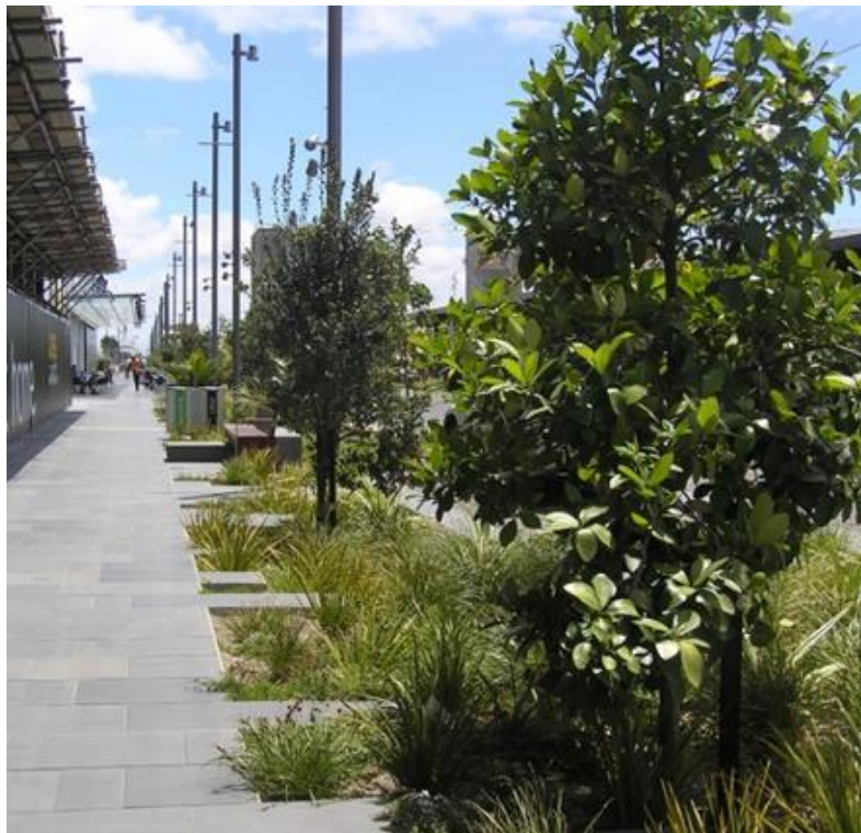
Photograph 1: Raingardens along Jellicoe St, Auckland Waterfront, as an example of modular design, each raingarden serves a small section of road (Photo: Sharleen Yalden).
