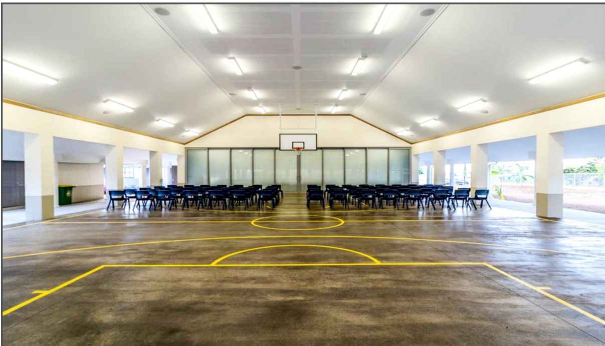
Figure 18 Latter-Day Saints Church in Lufilufi, Upolu. allowing for open cross-ventilation.
