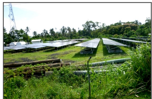
Figure 8 Samoa 0.5 MW Utility scale grid-connect solar Salelologa, Savai'i
