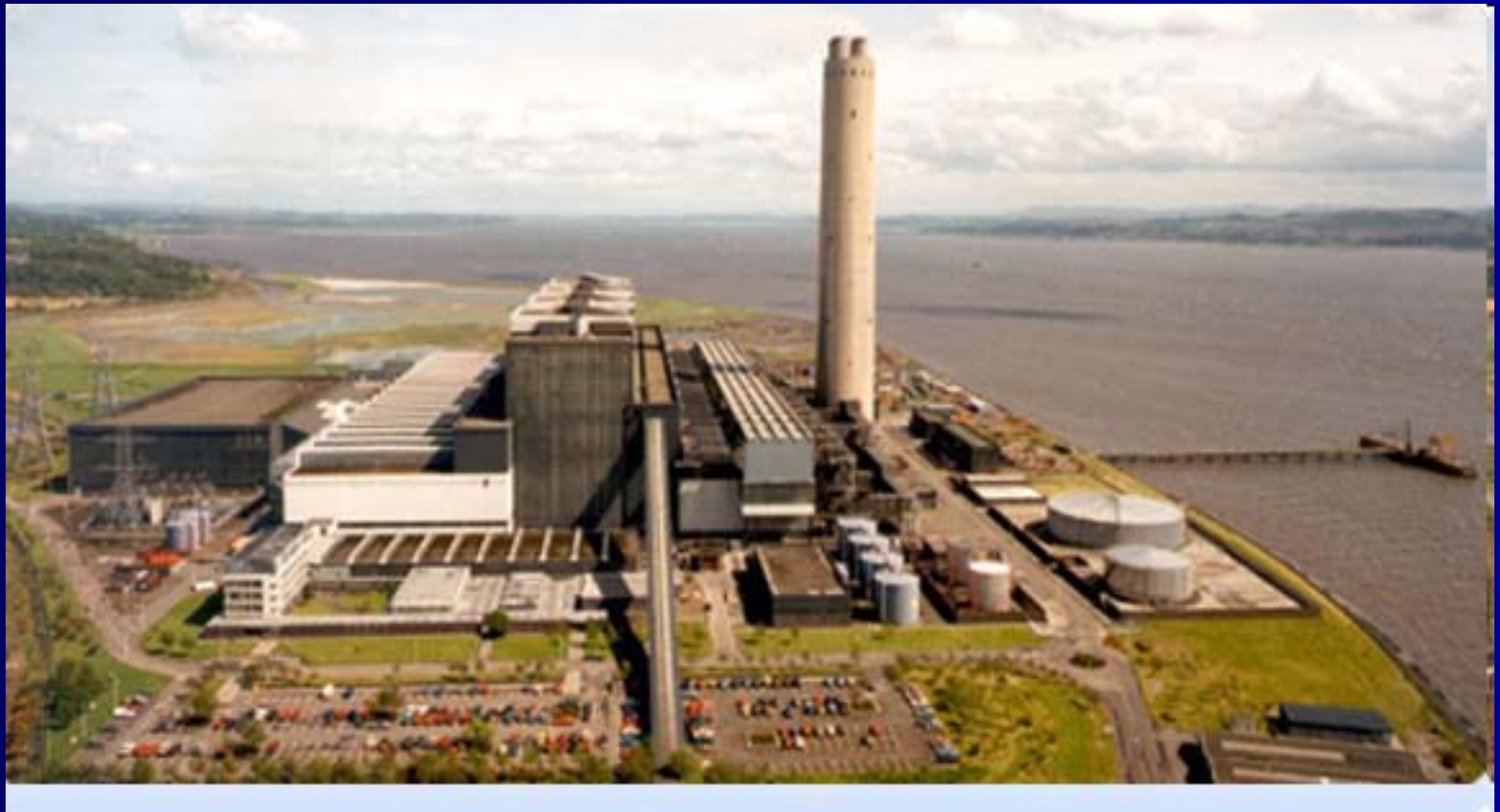
Green Energy biomass power station in West Fife, Scotland.
